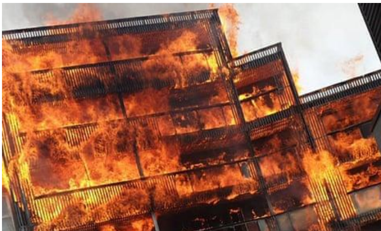
Figure 9: Barking Riverside fire - Entire section of balconies burning [24]
